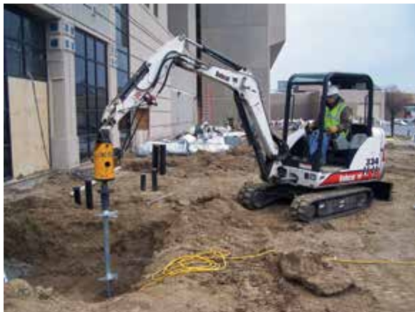
New construction helical pile installation
