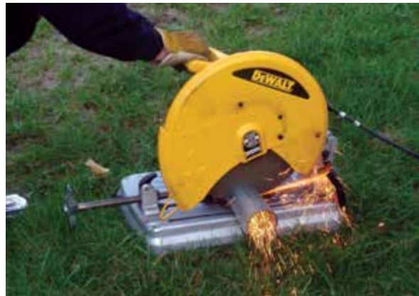
Figure 3.10.n Cutting pier tube to desired length with a chop saw
