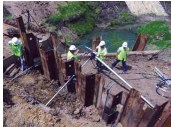
Helical tieback installation with hand-held equipment
