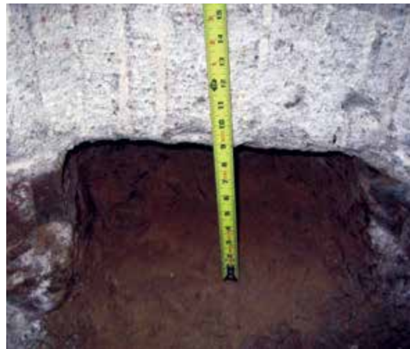
Figure 3.10.b3 Completed footing excavation and preparation; ready to position bracket
