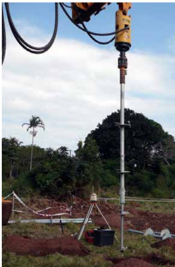
Figure 2.5.a Combination pile with HA175 stinger coupled immediately to 3.5" O.D. shaft
