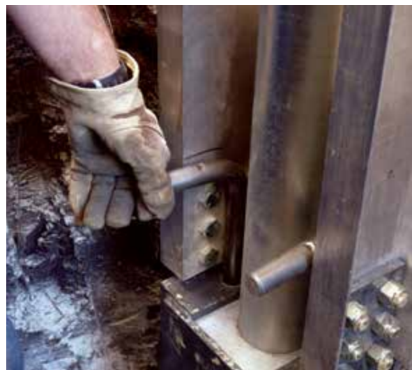
Figure 3.10.e2 PP288 drive stand secured to the bracket with L-pins
