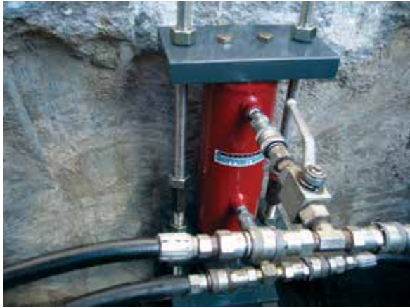
Figure 2.12.3.2.g Set hydraulic lift cylinders
