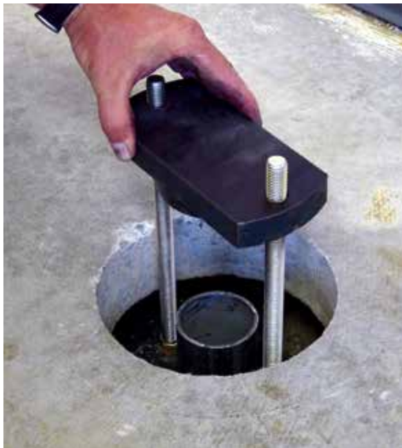
Figure 3.12.m Pier tube cut to length; pier cap placed
