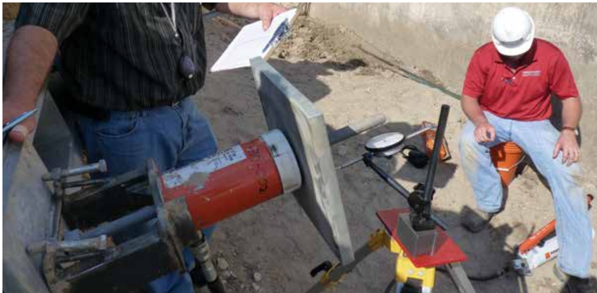
Figure 2.8.1.c Pre-tensioning helical tieback
