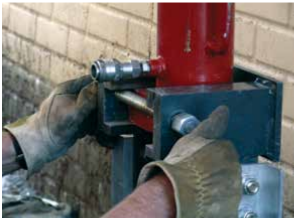
Figure 3.10.f2 Drive cylinder locked in position with coil rod and nuts
