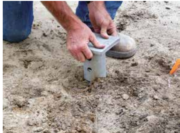
Figure 2.12.3.1.b Install new construction bracket
