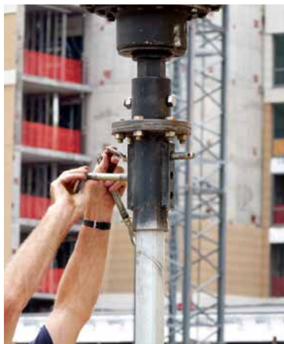
Figure 2.12.2.2.b Round shaft product adaptor
