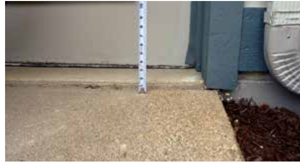
Figure 5.2.b2 After: Driveway lifted back to near original elevation
