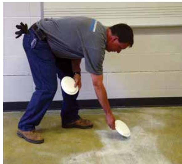
Figure 3.12.a Marking slab pier locations
