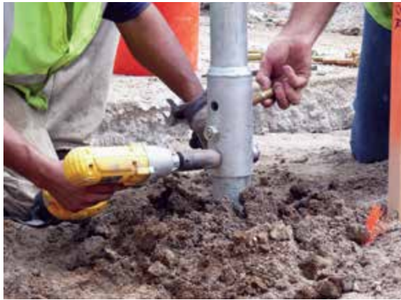
Figure 2.12.3.1.a Install coupler bolts
