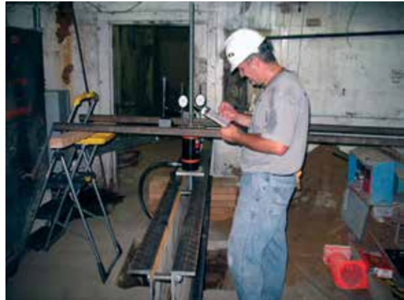
Figure 2.10.b2 Tension load test within basement
