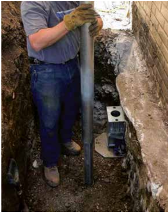
Figure 3.10.d1 Exterior sleeve slid over the starter tube
