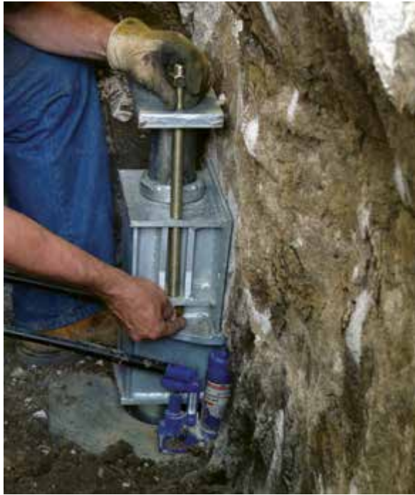
Figure 3.10.o1 Installation of pier cap plate with threaded rods and nuts
