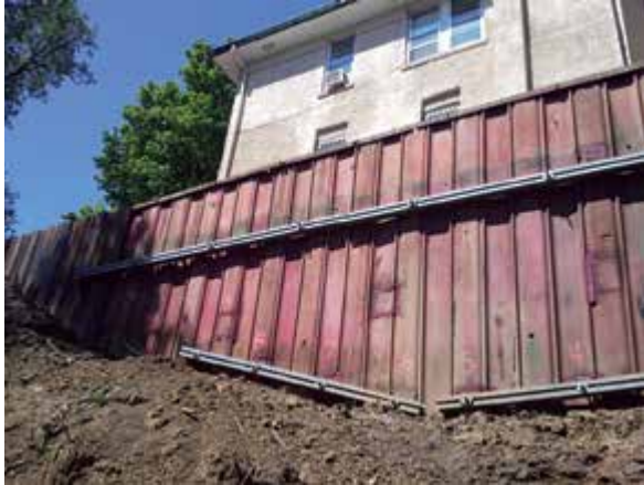
Figure 2.8.c1 Helical tiebacks stabilize sheet pile wall below historic home
