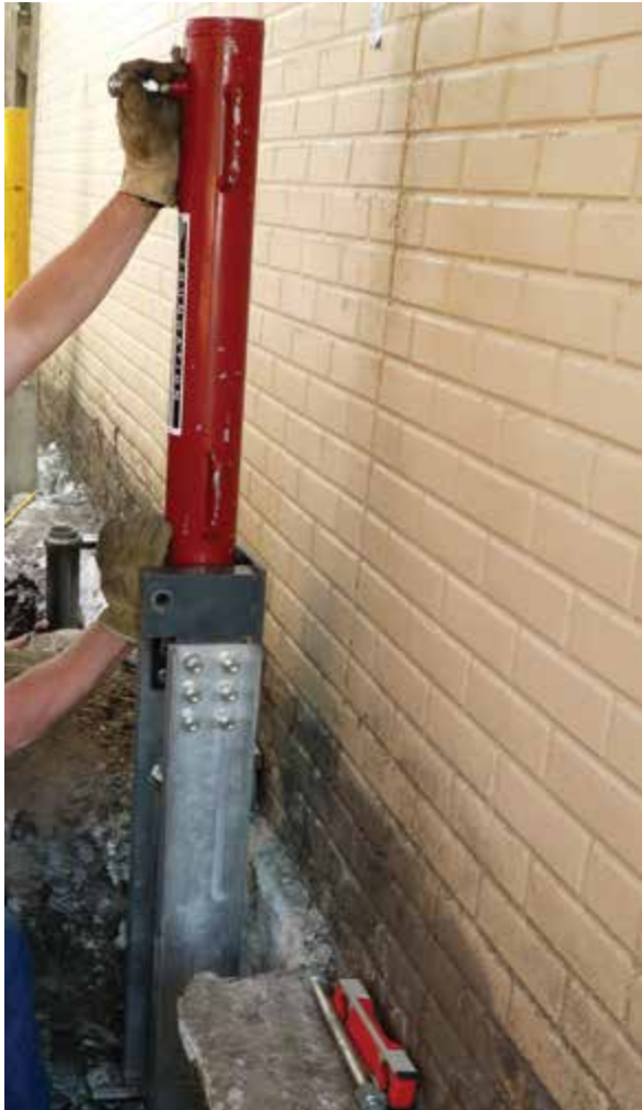
Figure 3.10.f1 Hydraulic drive cylinder placed within top fixture of drive stand
