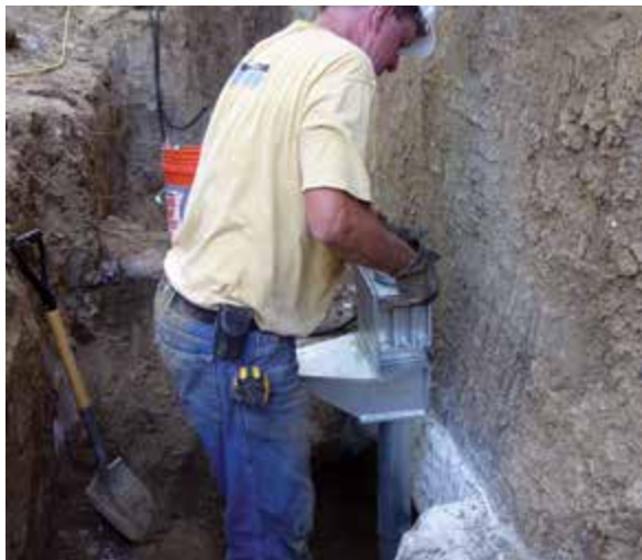
Figure 2.12.3.2.d Lower assembly over pile shaft
