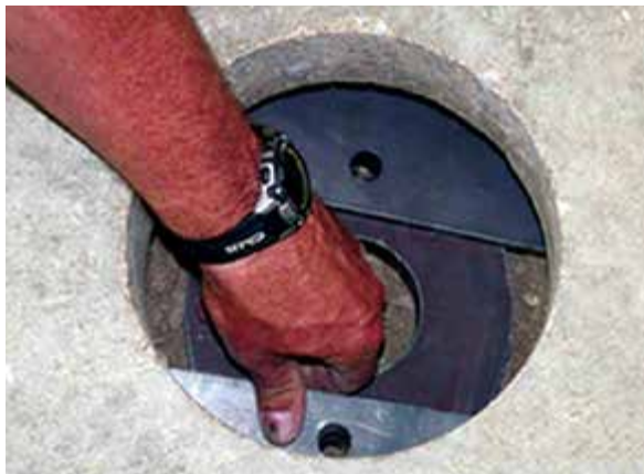
Figure 3.12.f Main plate and wing plates positioned and aligned beneath the slab
