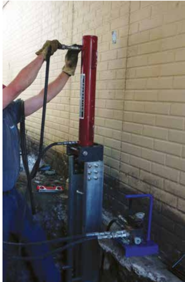
Figure 3.10.g Connect hydraulic hoses
