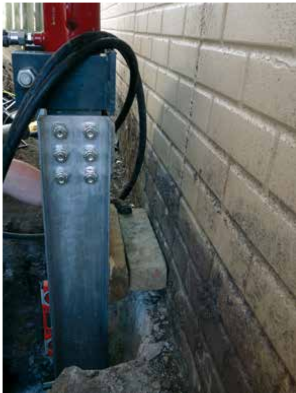
Figure 3.10.i Temporary wood cribbing used to set installation angle
