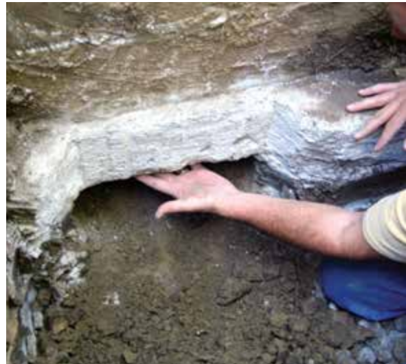
Figures 3.10.b2 Checking underside of footing for proper preparation
