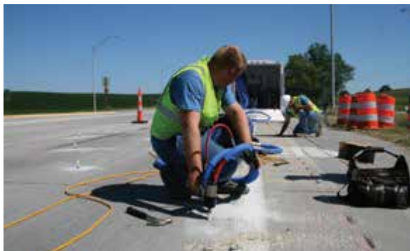
Figure 5.2.d2 Monitoring pavement lift with string lines
