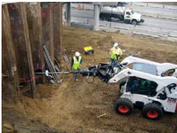
Sheet pile wall stabilization with helical tiebacks
