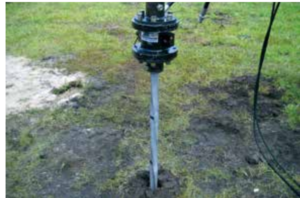
Figure 2.12.2.3.d Shaft twist
