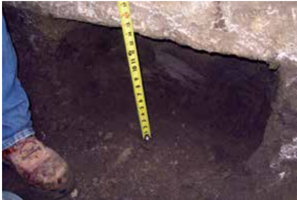
Figure 2.12.3.2.a Excavation at bracket
