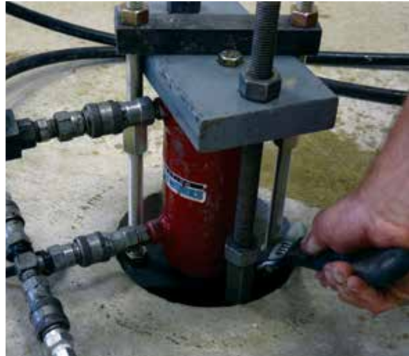
Figure 3.12.s Pier load locked off by tightening nuts on top of pier cap
