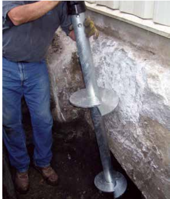
Figure 2.12.3.2.c Alignment of lead
