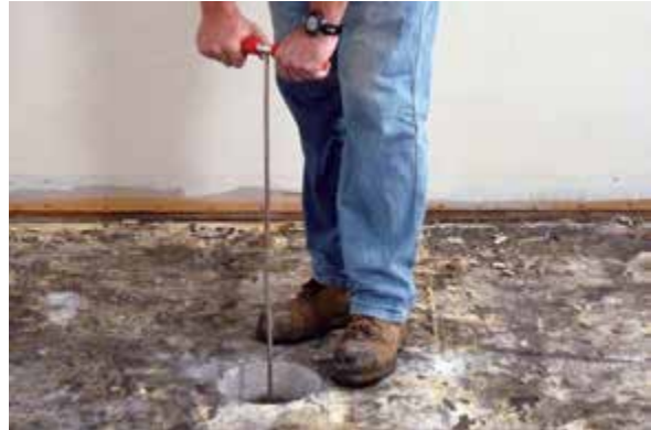
Figures 3.12.d Probing for utilities or obstructions
