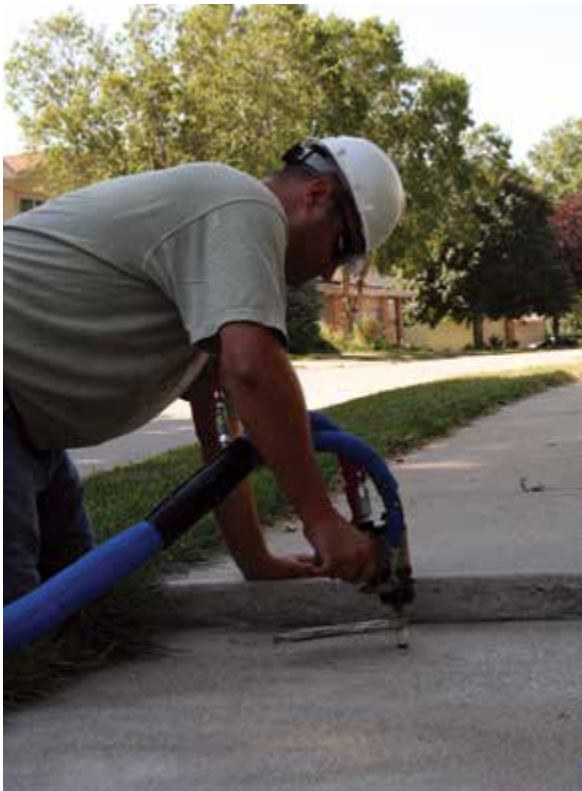
Figure 5.2.a PolyLEVEL foam injected to re-level faulted sidewalk sections
