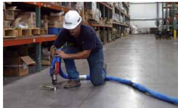
Figure 5.2.c PolyLEVEL stabilizes warehouse floor slab
