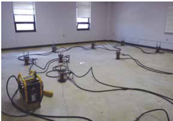
Figure 3.12.r Lift cylinders in series
