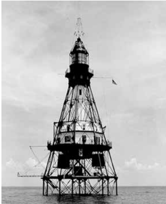
Lighthouse supported by helical pile foundations
