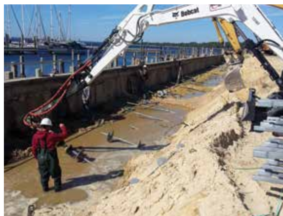
Figure 2.8.b Helical tiebacks stabilize marina seawall
