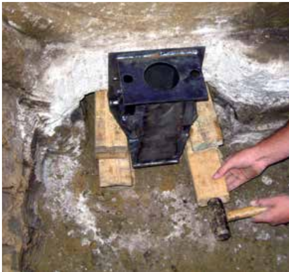
Figure 3.10.c1 Temporary bracket support with wood cribbing
