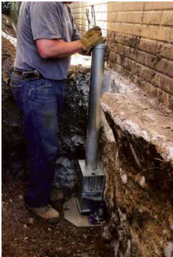
Figure 3.10.d2 Sleeve and starter inserted together through the bracket
