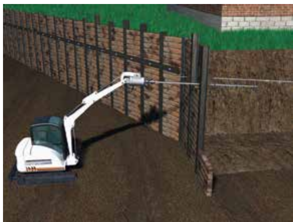
Figure 2.8.a1 Rendering of helical tieback installation for soldier pile and timber lagging wall
