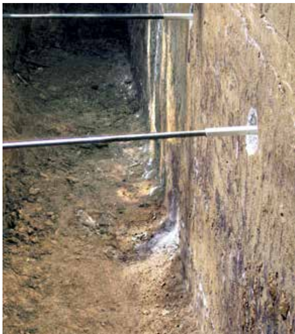
Figure 4.2.5.1.b2 After: Shear movement recovered and wall stabilized with Geo-Lock anchors
