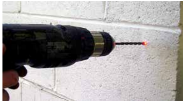
Figure 3.10.r Benchmark established with a shallow hole drilled into the concrete block
