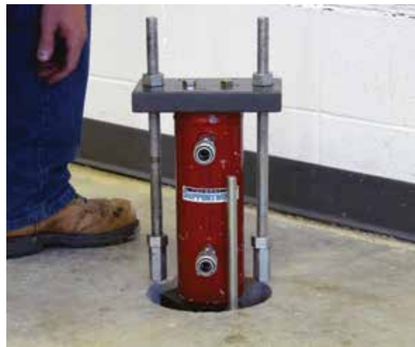
Figure 3.12.o Lift cylinder assembly set on pier cap
