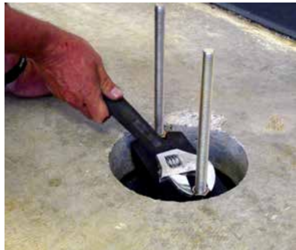
Figure 3.12.n Lightly tighten pier cap down onto pier tube
