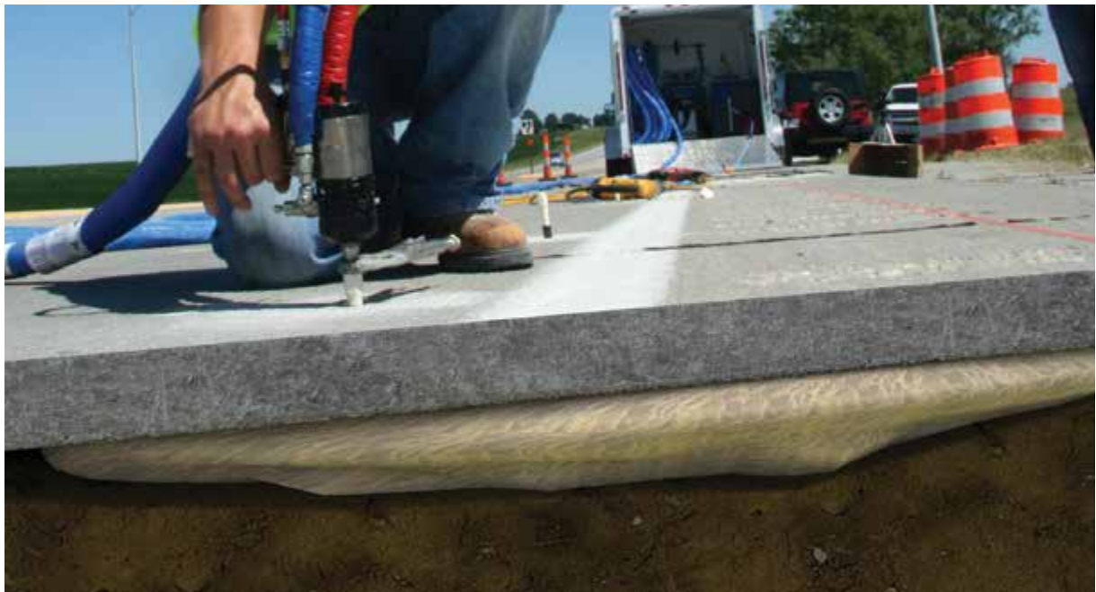
Figure 5.1.a Rendering of PolyLEVEL foam injection beneath concrete pavement
