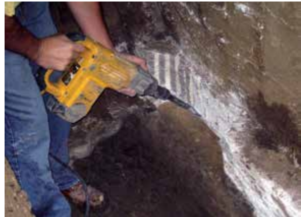
Figure 3.10.b1 Smoothing the vertical and horizontal bearing surfaces with a chipping hammer
