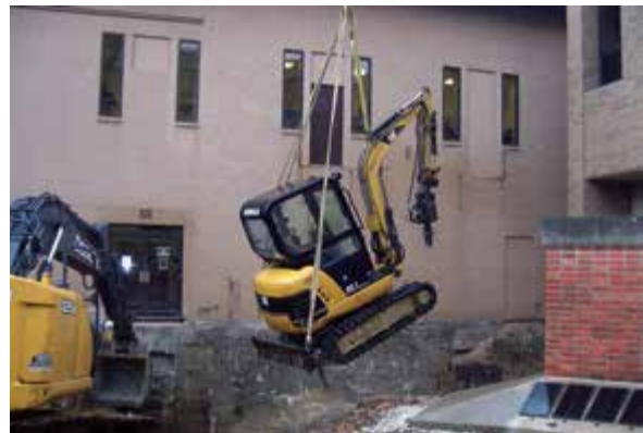
Figure 2.4.a2 Mini-excavator lowered by crane into excavation to install helical tiebacks
