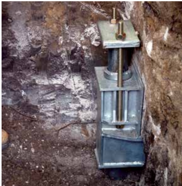
Figure 3.10.o2 PP288 bracket ready for lift cylinder assembly
