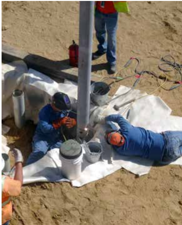
Figure 2.3.2.1.f FSI HP700 with complete joint penetration welds between sections
