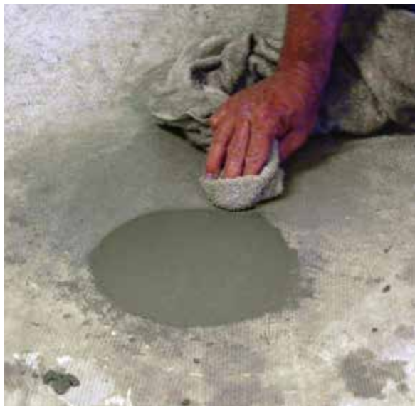
Figure 3.12.v Finishing concrete
