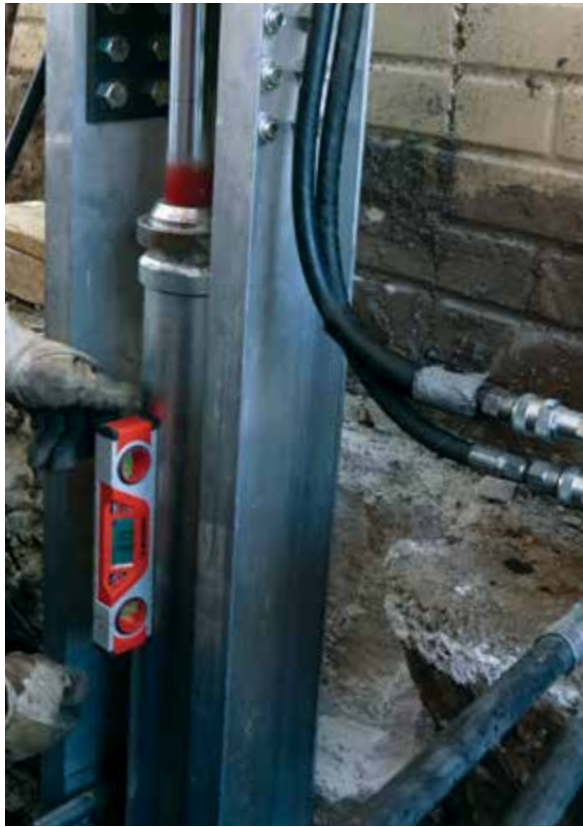
Figure 3.10.h Checking drive stand alignment with digital level
