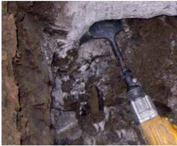
Figure 3.10.a Removing soil from beneath the footing with a chisel attachment
