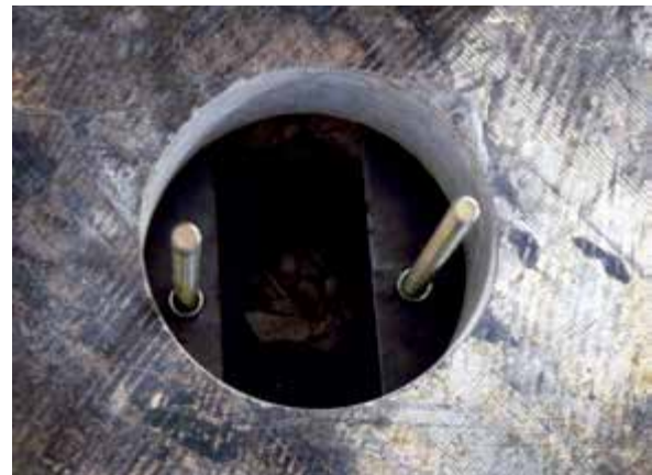
Figure 3.12.g Threaded rods installed
