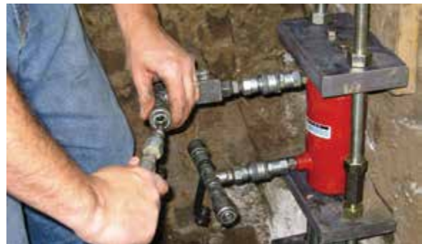
Figure 3.10.p1 Connection of lift cylinder assembly
