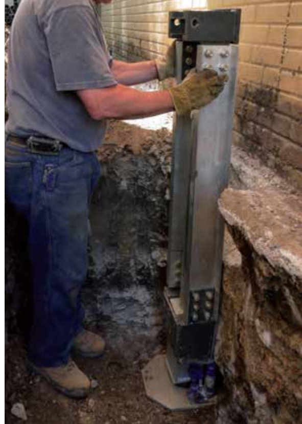
Figure 3.10.e1 Drive stand for PP288 push pier system fitted to the bracket
