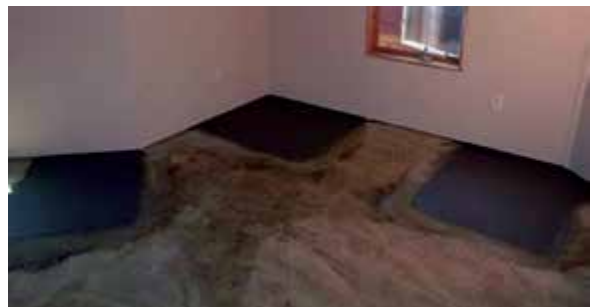
Figure 3.10.t Concrete placement at interior pier locations
