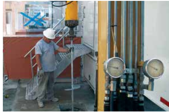
Figure 2.12.2.3.a2 Monitoring pressure gauges while installing square shaft helical anchor
