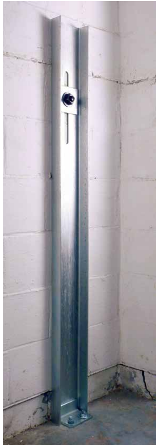
Figure 4.2.5.1.b3 Geo-Lock channel anchor system installed to prevent shear movement
