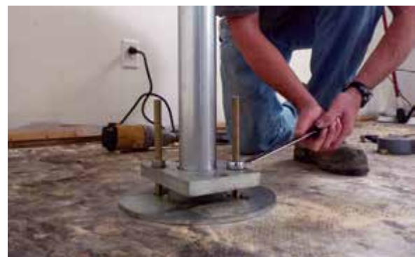
Figure 3.12.i Slab pier drive adaptor installed
