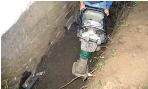
Figure 2.12.3.2.h Backfill and compact soil
