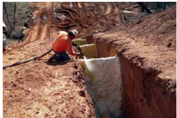
Figure 5.2.e Placement of polyurethane foam trench breaks
