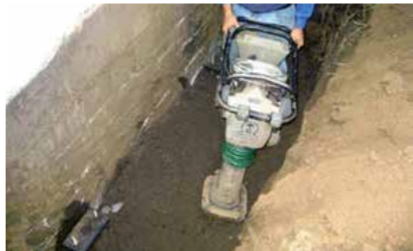
Figure 3.10.s Backfill excavations and compact soil
