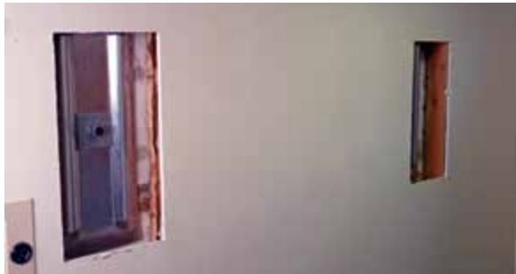
Figure 4.2.5.2.a1 Geo-Lock wall anchor installed through drywall penetration and between wood studs
