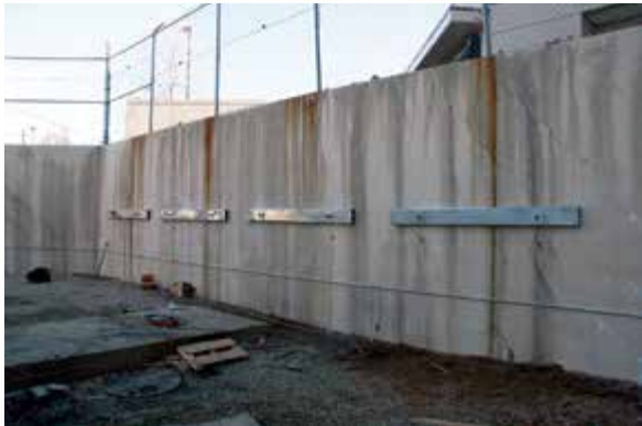
Figure 2.8.c2 Helical tiebacks and tube steel walers stabilize concrete retaining wall
