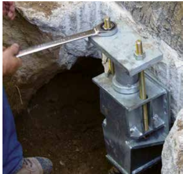
Figure 2.12.3.2.f Install cap plate and rods
