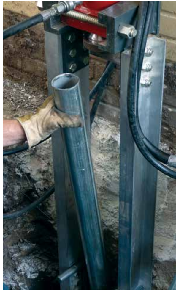
Figure 3.10.j Installing PP288 push pier tube
