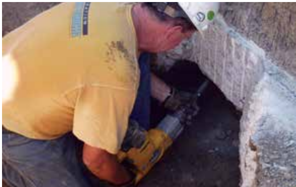
Figure 2.12.3.2.b Footing preparation
