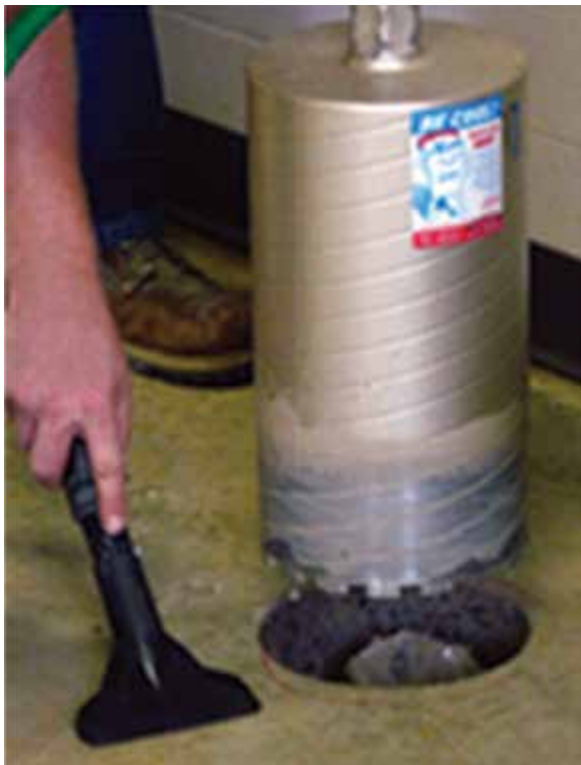
Figure 3.12.c Concrete coring
