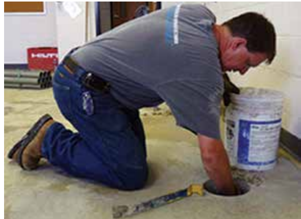
Figure 3.12.e Excavating beneath the slab
