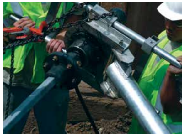
Figure 2.12.2.2.c Square shaft adaptor
