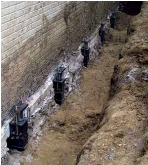
Figure 3.10.q System locked off; pier installation complete
