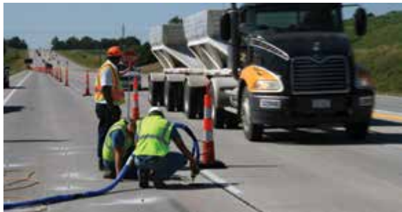
Figure 5.2.d1 PolyLEVEL injection while maintaining an open lane for traffic
