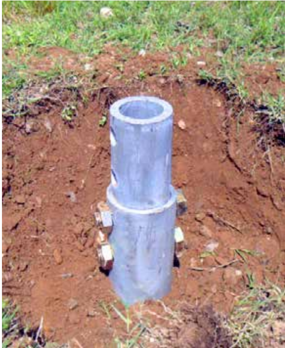
Figure 2.3.2.1.b Internal detached coupler detail of FSI HP450
