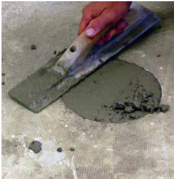
Figure 3.12.u Patching holes at pier locations
