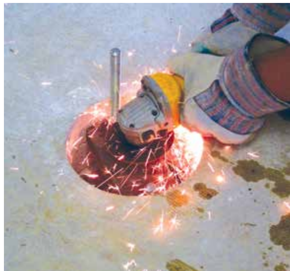
Figure 3.12.t Cutting the threaded rods
