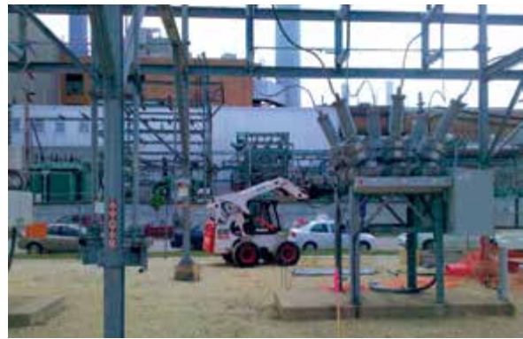
Figure 2.4.a1 Skid steer installing helical piles within limited space at a substation
