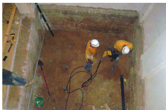
Figure 2.4.a3 Helical piles installed with hand-held equipment to support new elevator within existing school
