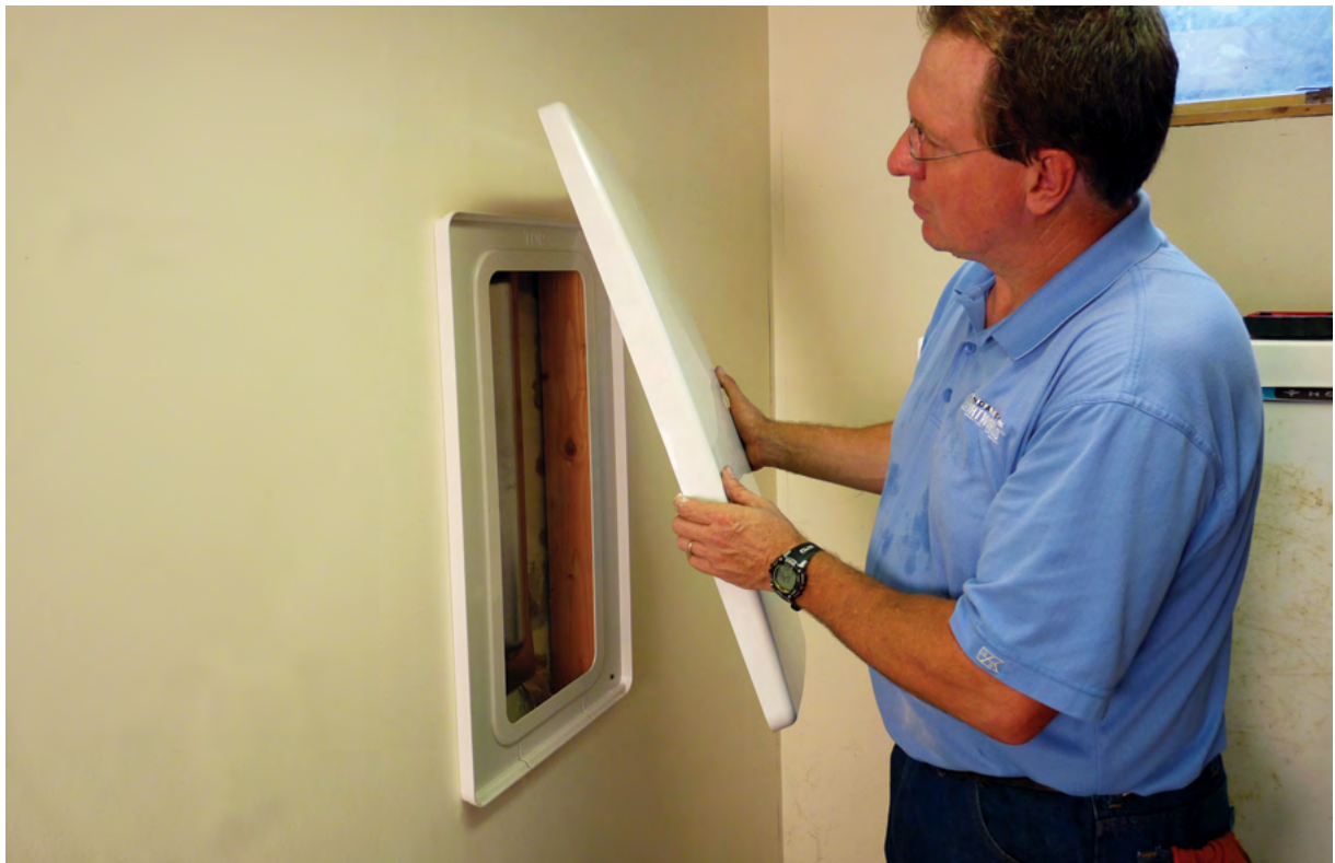
Figure 4.2.5.2.a3 Hide-A-Way wall anchor cover installed
