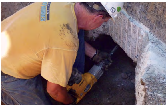
Figure 2.12.3.2.b Footing preparation
