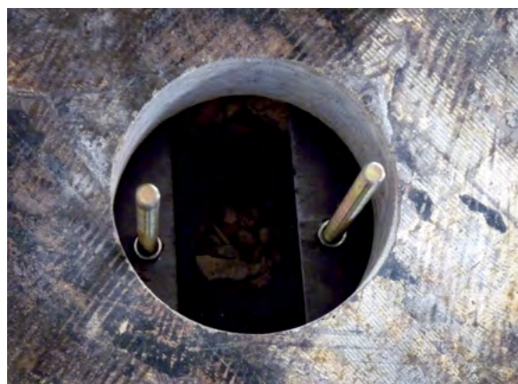
Figure 3.12.g Threaded rods installed
