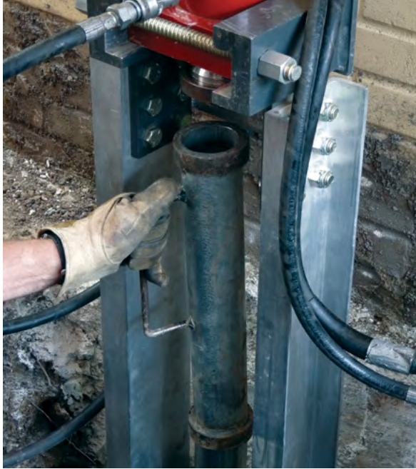
Figure 3.10.k Driving tube tool set in place for second stage of push
