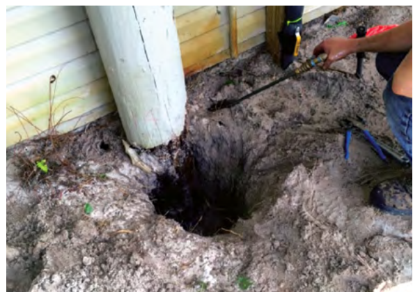
Figure 5.2.f PolyLEVEL resin stabilizes loose sand to prevent undermining of slab during column repair
