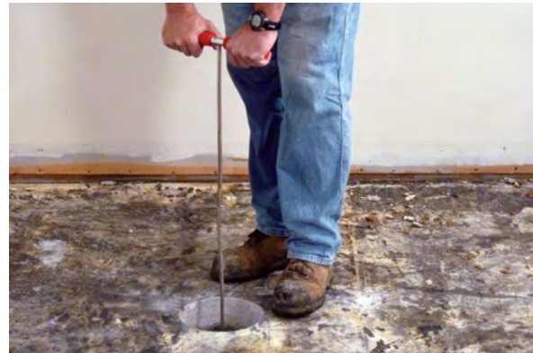
Figures 3.12.d Probing for utilities or obstructions
