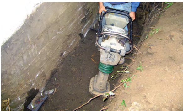
Figure 2.12.3.2.h Backfill and compact soil
