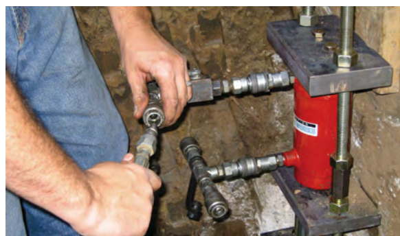
Figure 3.10.p1 Connection of lift cylinder assembly
