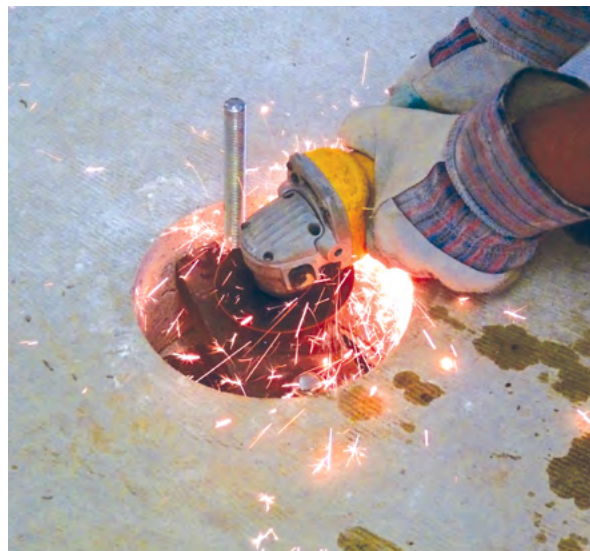
Figure 3.12.t Cutting the threaded rods
