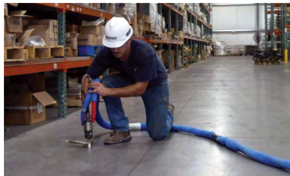
Figure 5.2.c PolyLEVEL stabilizes warehouse floor slab
