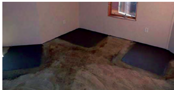
Figure 3.10.t Concrete placement at interior pier locations
