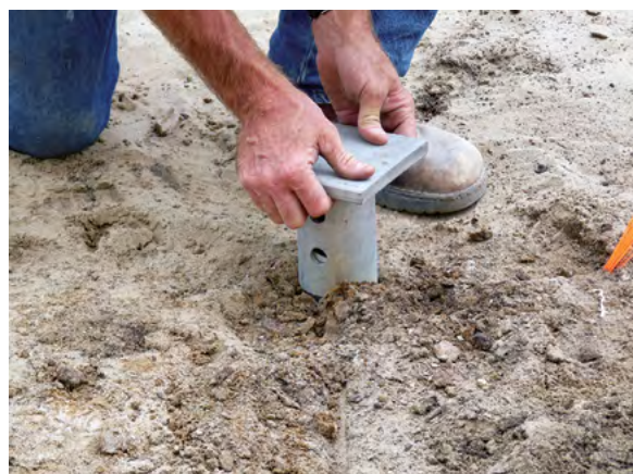
Figure 2.12.3.1.b Install new construction bracket
