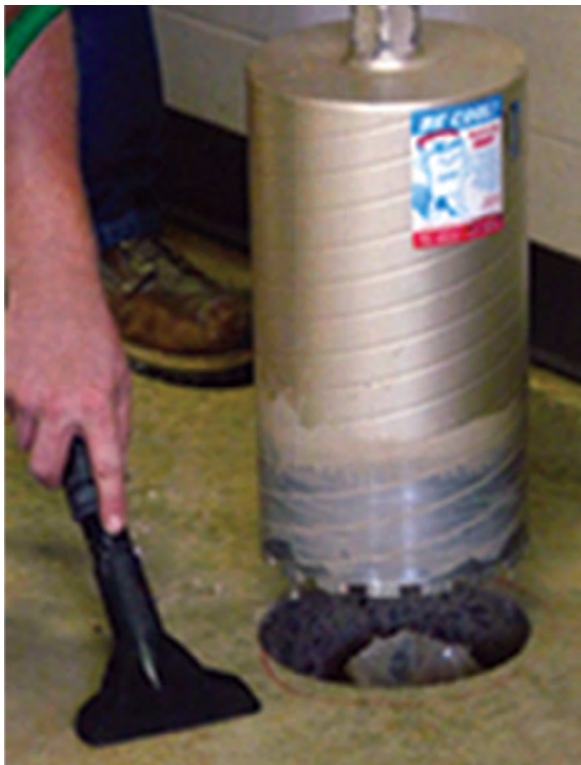
Figure 3.12.c Concrete coring
