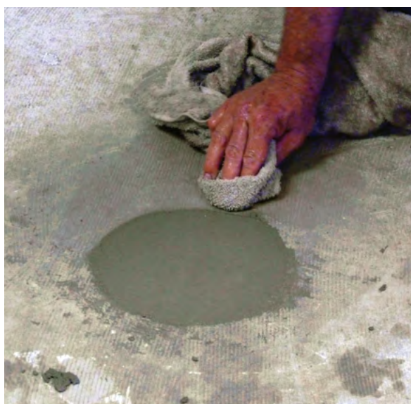
Figure 3.12.v Finishing concrete
