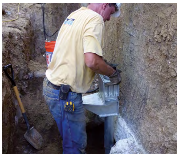
Figure 2.12.3.2.d Lower assembly over pile shaft
