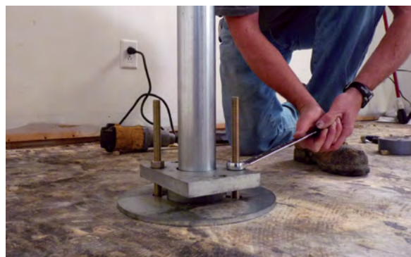
Figure 3.12.i Slab pier drive adaptor installed
