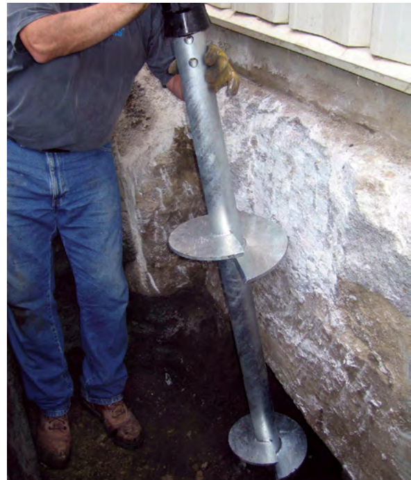
Figure 2.12.3.2.c Alignment of lead
