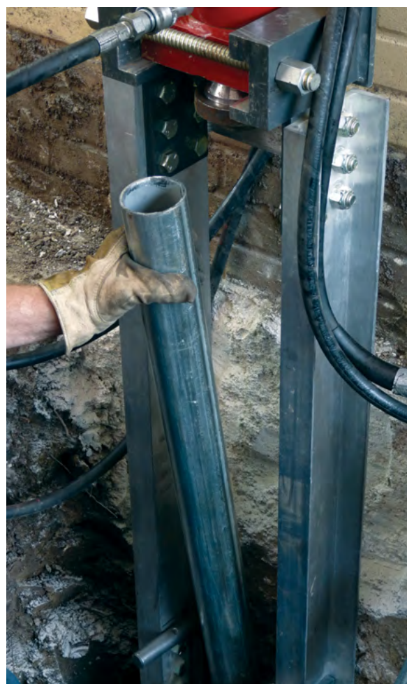
Figure 3.10.j Installing PP288 push pier tube
