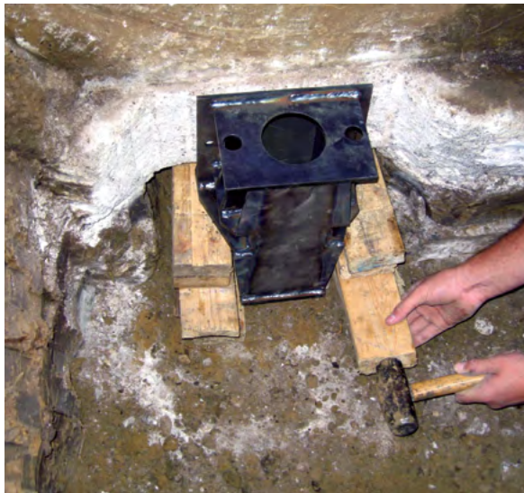
Figure 3.10.c1 Temporary bracket support with wood cribbing
