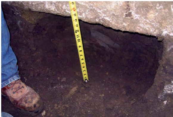
Figure 2.12.3.2.a Excavation at bracket
