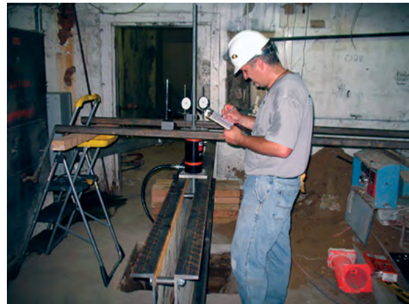
Figure 2.10.b2 Tension load test within basement
