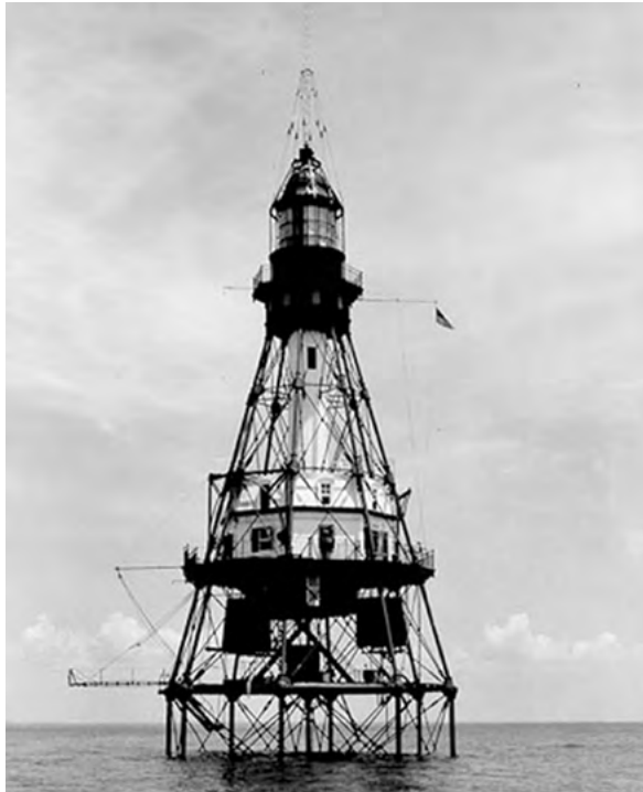
Lighthouse supported by helical pile foundations
