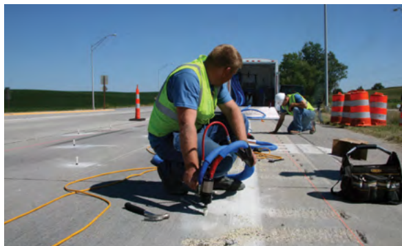
Figure 5.2.d2 Monitoring pavement lift with string lines
