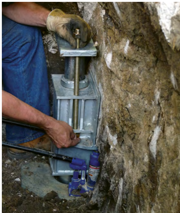
Figure 3.10.o1 Installation of pier cap plate with threaded rods and nuts
