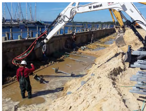
Figure 2.8.b Helical tiebacks stabilize marina seawall
