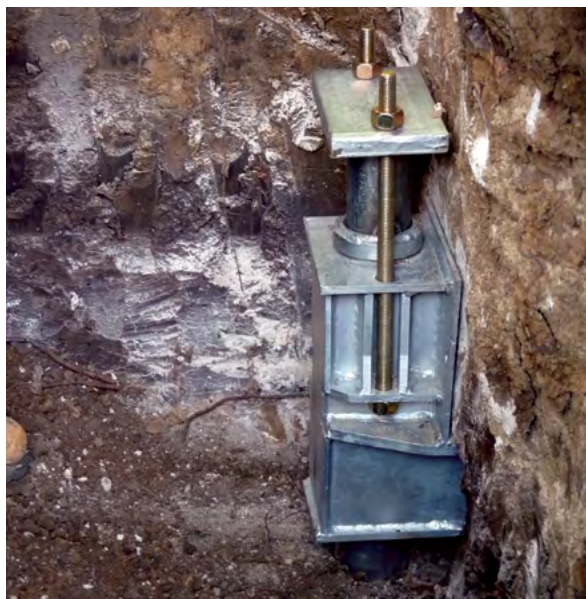
Figure 3.10.o2 PP288 bracket ready for lift cylinder assembly
