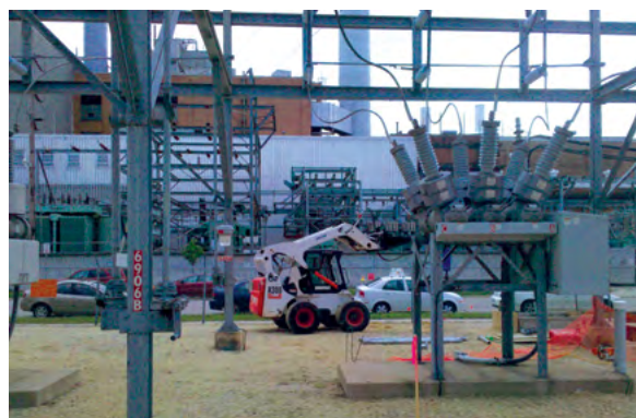
Figure 2.4.a1 Skid steer installing helical piles within limited space at a substation
