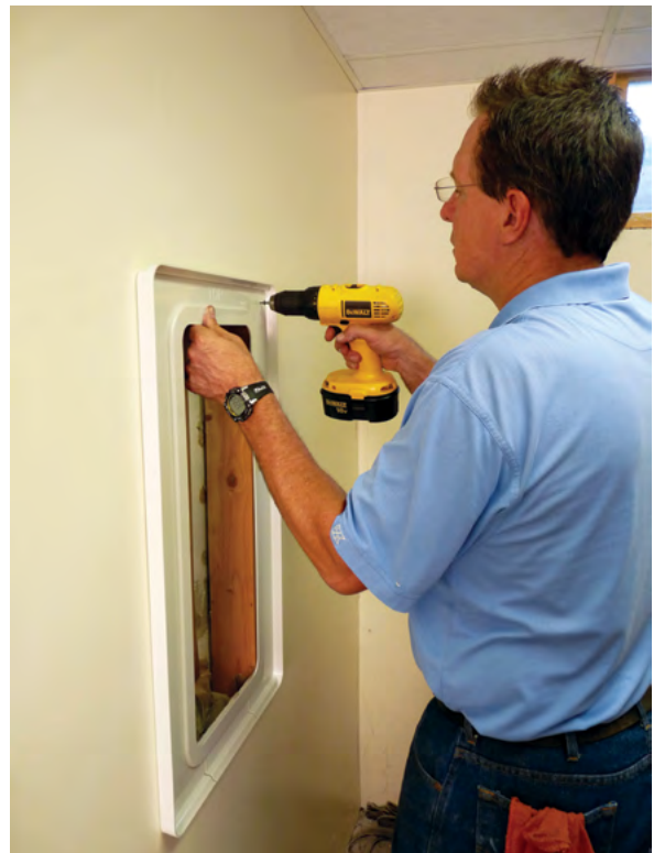
Figure 4.2.5.2.a2 Frame for Hide-A-Way cover installed around drywall opening
