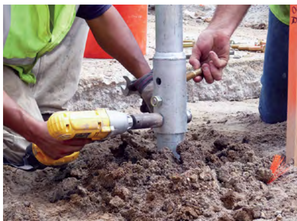
Figure 2.12.3.1.a Install coupler bolts
