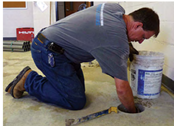
Figure 3.12.e Excavating beneath the slab
