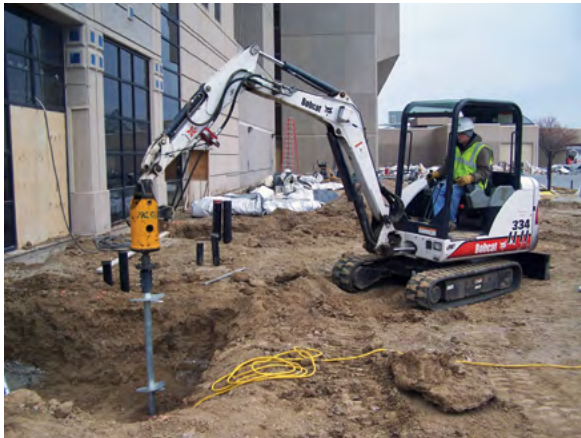
New construction helical pile installation
