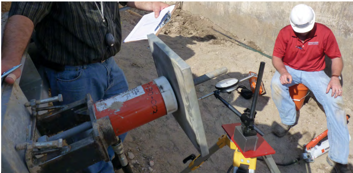
Figure 2.8.1.c Pre-tensioning helical tieback
