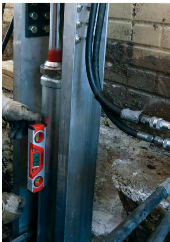
Figure 3.10.h Checking drive stand alignment with digital level
