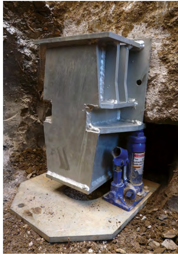
Figure 3.10.c2 Bracket RAYser™ support system
