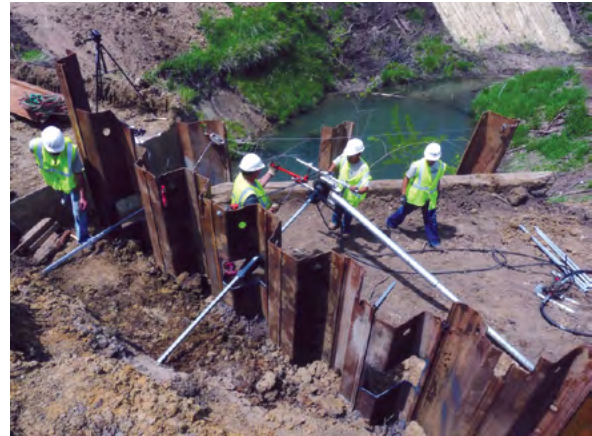
Helical tieback installation with hand-held equipment
