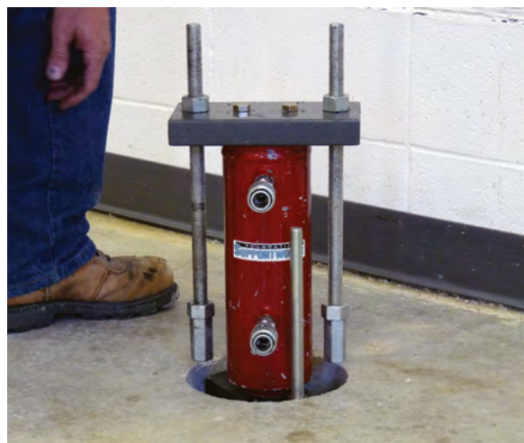
Figure 3.12.o Lift cylinder assembly set on pier cap
