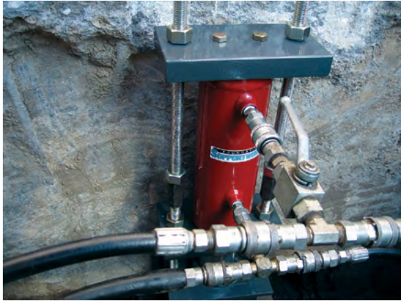
Figure 2.12.3.2.g Set hydraulic lift cylinders
