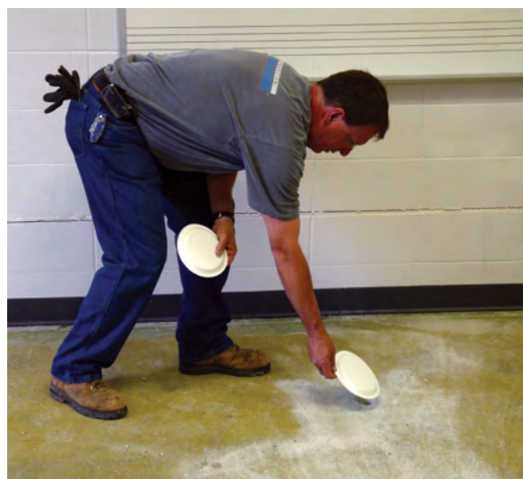
Figure 3.12.a Marking slab pier locations
