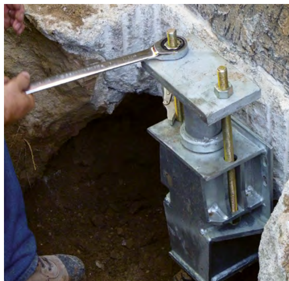
Figure 2.12.3.2.f Install cap plate and rods
