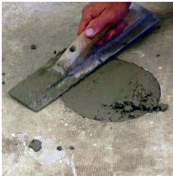
Figure 3.12.u Patching holes at pier locations
