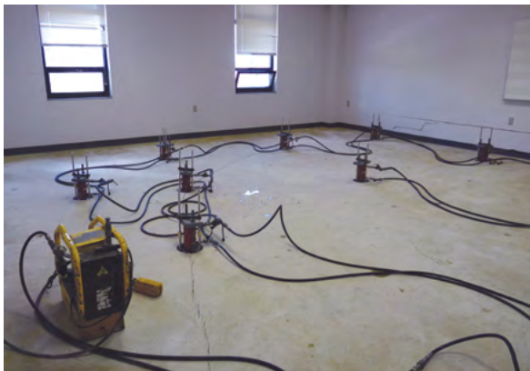
Figure 3.12.r Lift cylinders in series
