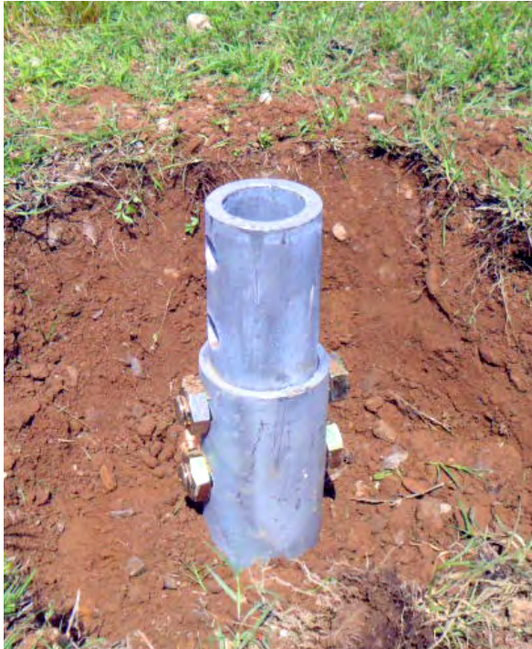
Figure 2.3.2.1.b Internal detached coupler detail of FSI HP450
