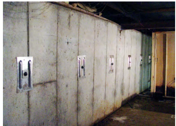
Figure 4.2.5.1.a2 After: Wall is immediately returned to original straight position after backfill soil is removed and Geo-Lock anchors installed
