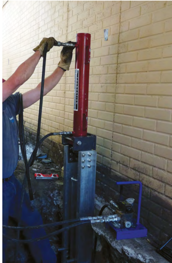
Figure 3.10.g Connect hydraulic hoses
