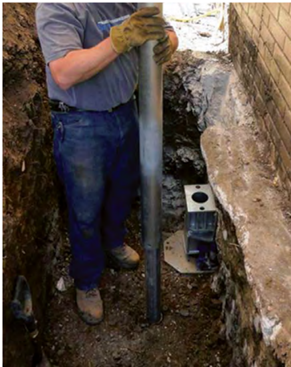
Figure 3.10.d1 Exterior sleeve slid over the starter tube
