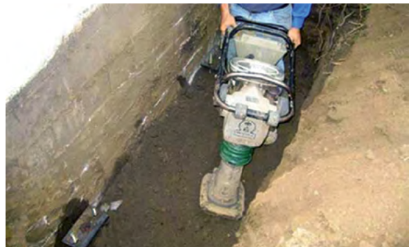
Figure 3.10.s Backfill excavations and compact soil
