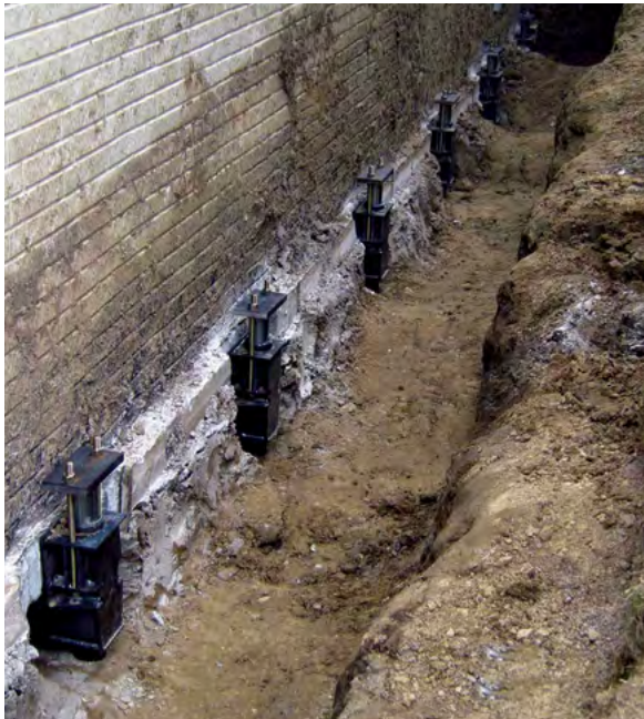
Figure 3.10.q System locked off; pier installation complete
